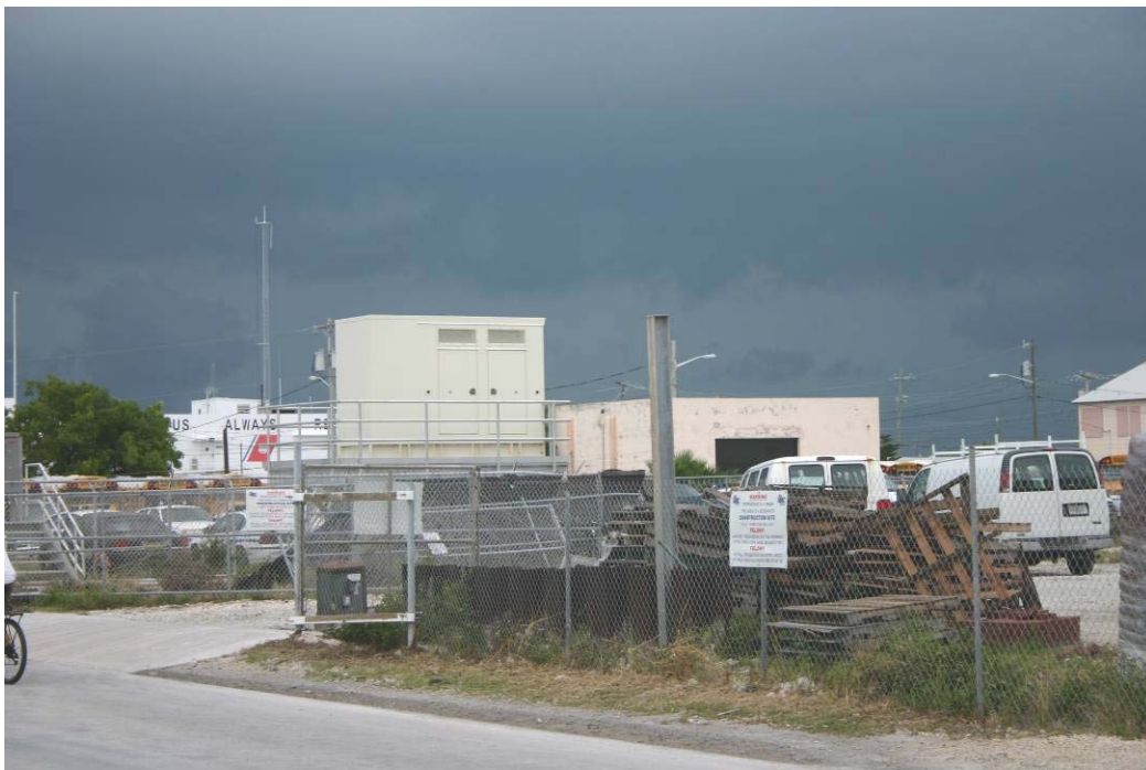
Top Photograph: Deteriorated Buildings and Storage Yard, Trumbo Road Area (Source: City of Key West, 2009); Bottom Photograph: Storage Area, Trumbo Road Area (Source: City of Key West, 2009)
