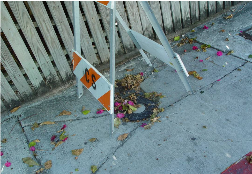
Top Photograph: Antiquated Land Uses, Dilapidated CES Substation Building (Source: City of Key West, 2009); Bottom Photograph: Typical Broken Sidewalk (Source: City of Key West, 2009)
